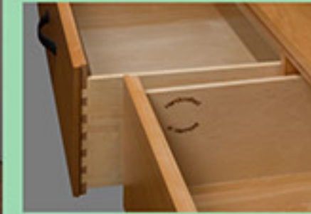
Dovetail Drawer Construction
