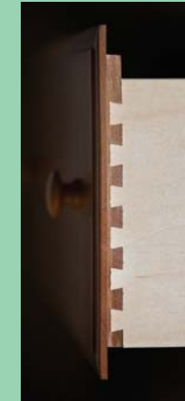
Dovetail Drawer Construction
